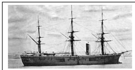
(Right above: *The photograph of the hybrid (sail and steam) armoured corvette HMS 'Penelope' is from the Wikipedia web-site.*)
