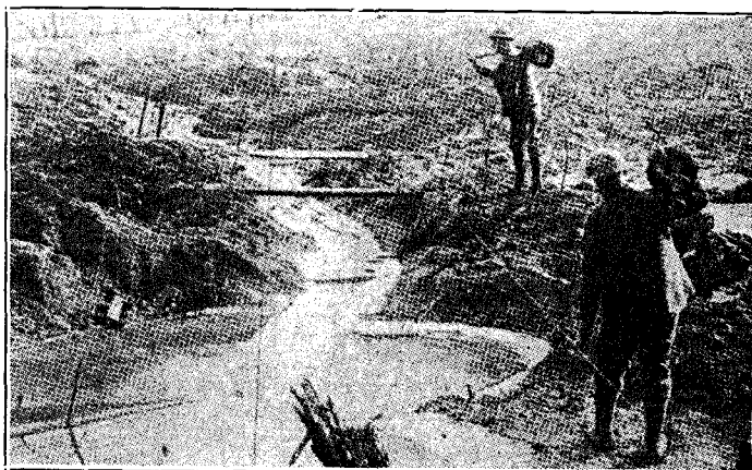
A Trench in France during the Winter of 1916-1917.
