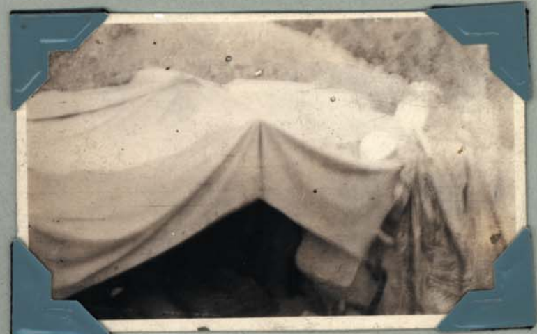
Officer's dugout with rubber sheet as covering. 1st. Nfld. Regt., Suvla Bay.
